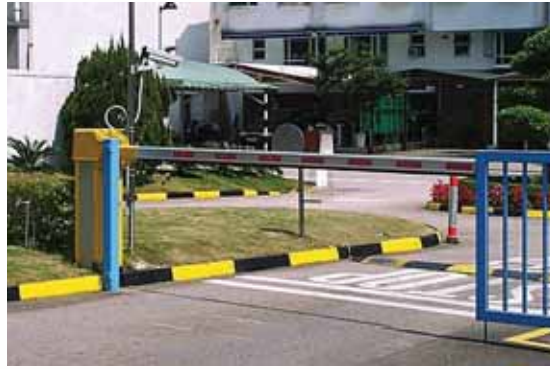
▼ Carpark Barrier System
